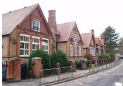
Unsympathetic railings outside the school
