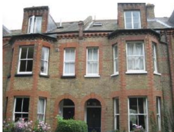
Marian & Georgiana Villas, nos. 35-37, building of townscape merit
